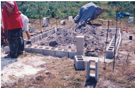
Denman Road Repeater Bldg
